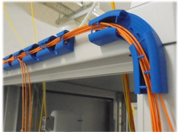
Routing the optical fiber cables on the side of a rack
